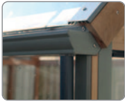
Guttering and downpipes
