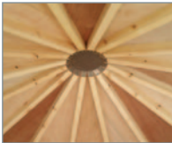
Internal roof structure
