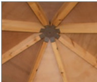
Internal roof structure
